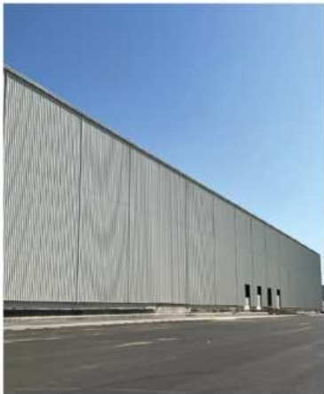
16 m High Refrigerator
