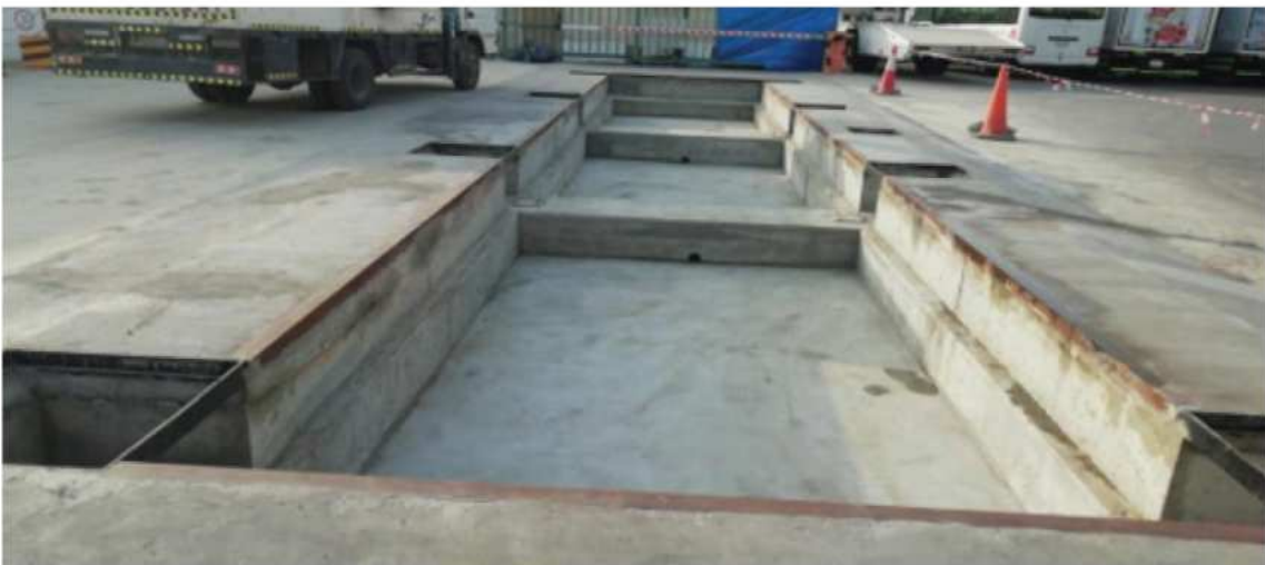
Ministry of Water Project Buraydah city
